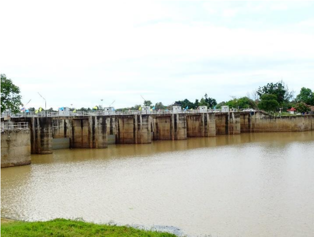
Fig. 3. The Rasi Salai Dam
