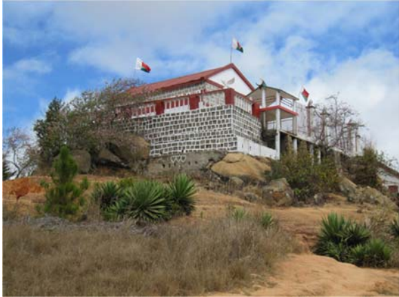
Main building of doany
