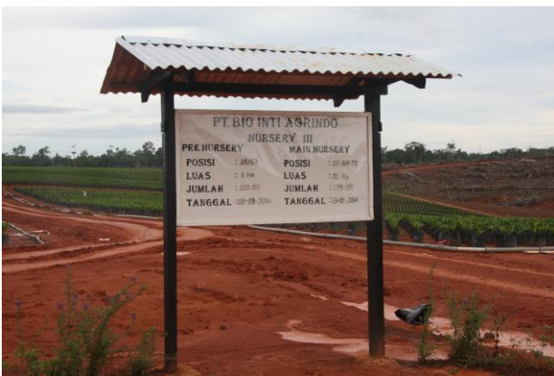
Preparation for a palm oil plantation; this plantation will open over more or less all of the 36.000 Ha
